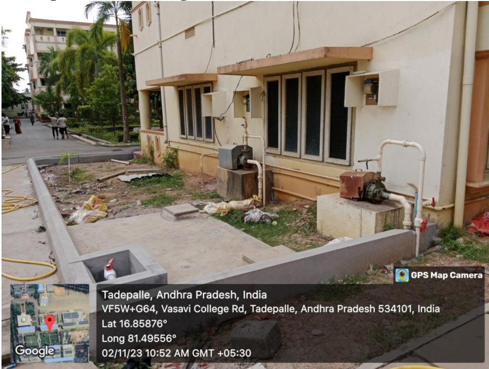
RO waste water to saved in tank for supplying water to washrooms and labs
