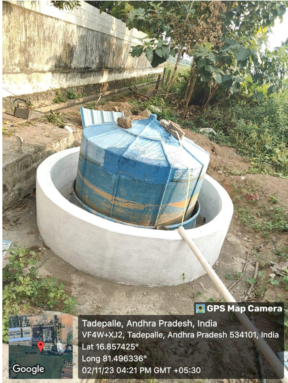
Bio gas plant
